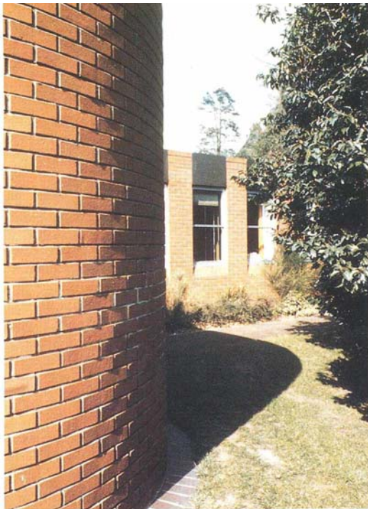
Figure 1 Faceting due to difference of arc and chord
