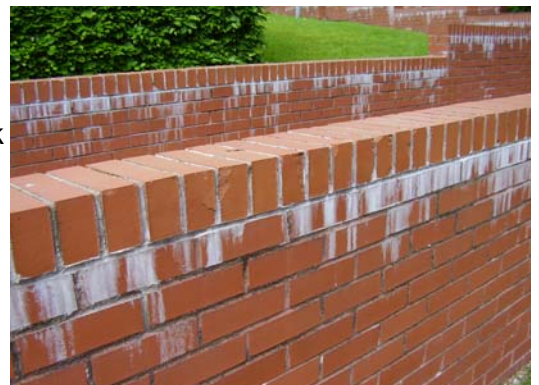
Both photos show omission of appropriate damp-proofing
