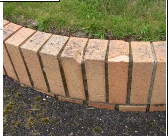
Both photos show omission of appropriate damp-proofing
