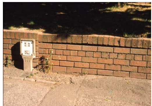
Capping lifts clear due to pressure
