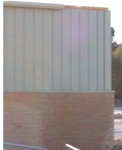
Saturation caused by missing guttering
