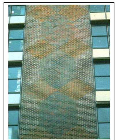
The effect that a different mortar mix can have on finished brickwork.
