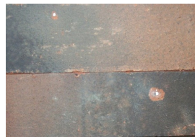
Expanded lime particles – noticeable on a colour sprayed surface
