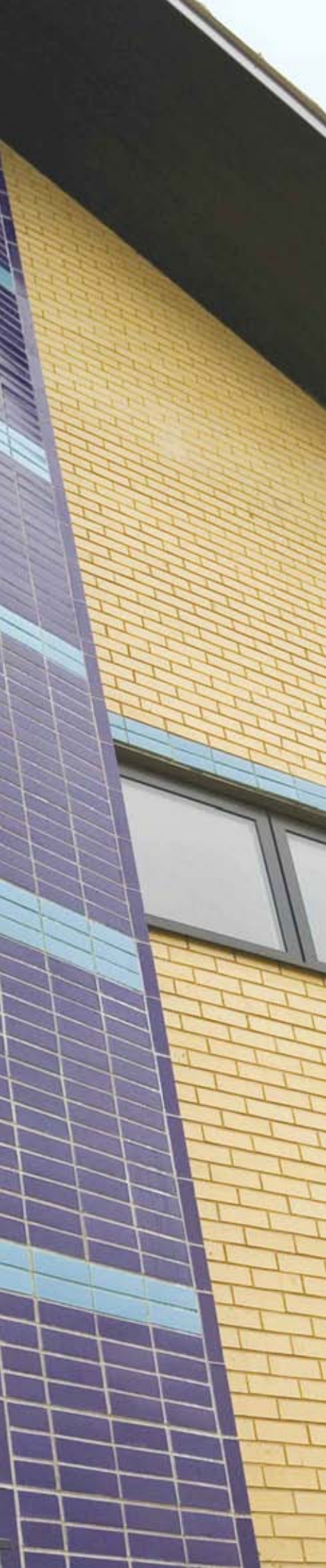
Private Housing, Kingston-upon-Hull | Blue Glazed Bricks
