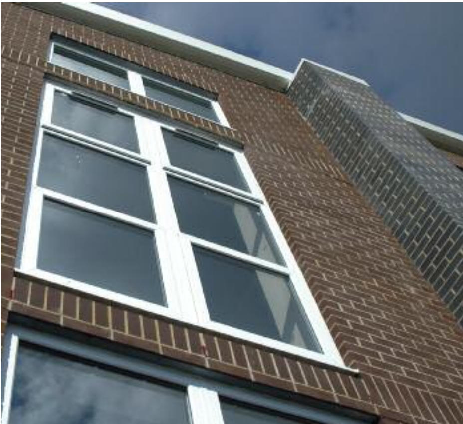
School, Shoreham, West Sussex | Holbrook Sandfaced Brown with Staffordshire Slate Blue Smooth
