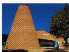
Best Structural Use of Brick World of Glass Museum, St Helens Architect: Geoffrey Reid Associates Structural Engineers: Building Design Practice Brickwork Contractor: Lightburn Construction (Leigh) Ltd
